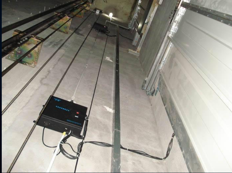
→ 竖直通道电力电缆敷设
